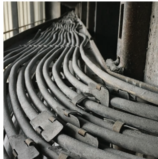
Examples of improper cable routing without cleats.
