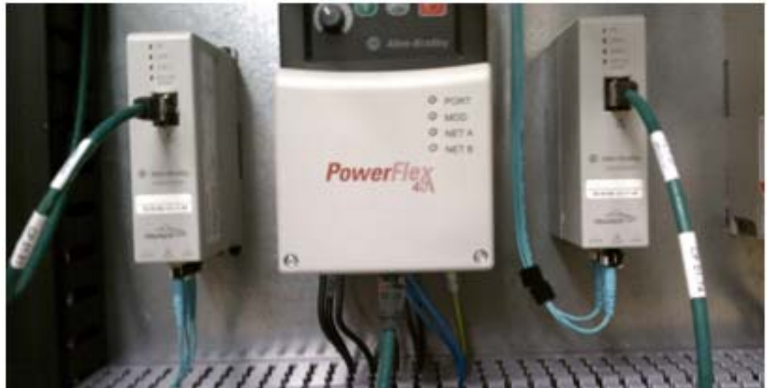
Figure 5 Sample Device-Level Fiber Optic Deployment
