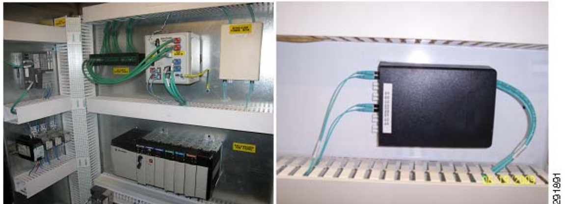
Figure 9 Sample Control Panel Fiber Optic Deployment
